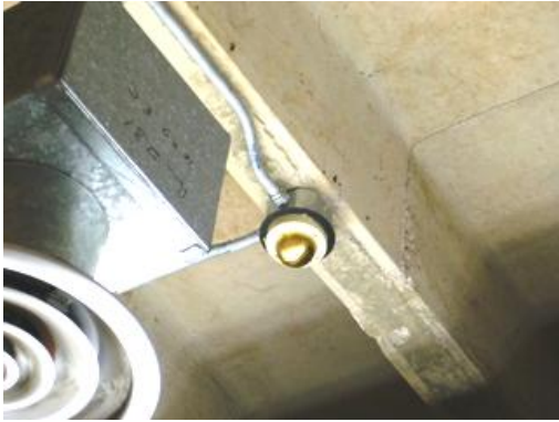
Figure 7. – Fixed temperature and ROR detector.
