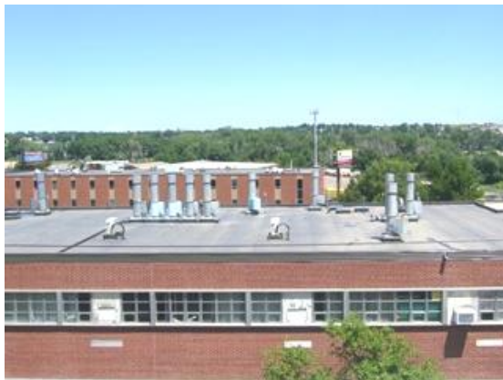
Figure 9. – Science Building Roof
