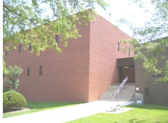
Figure 4. – EP Building – North Façade with second floor entry above grade plane.
